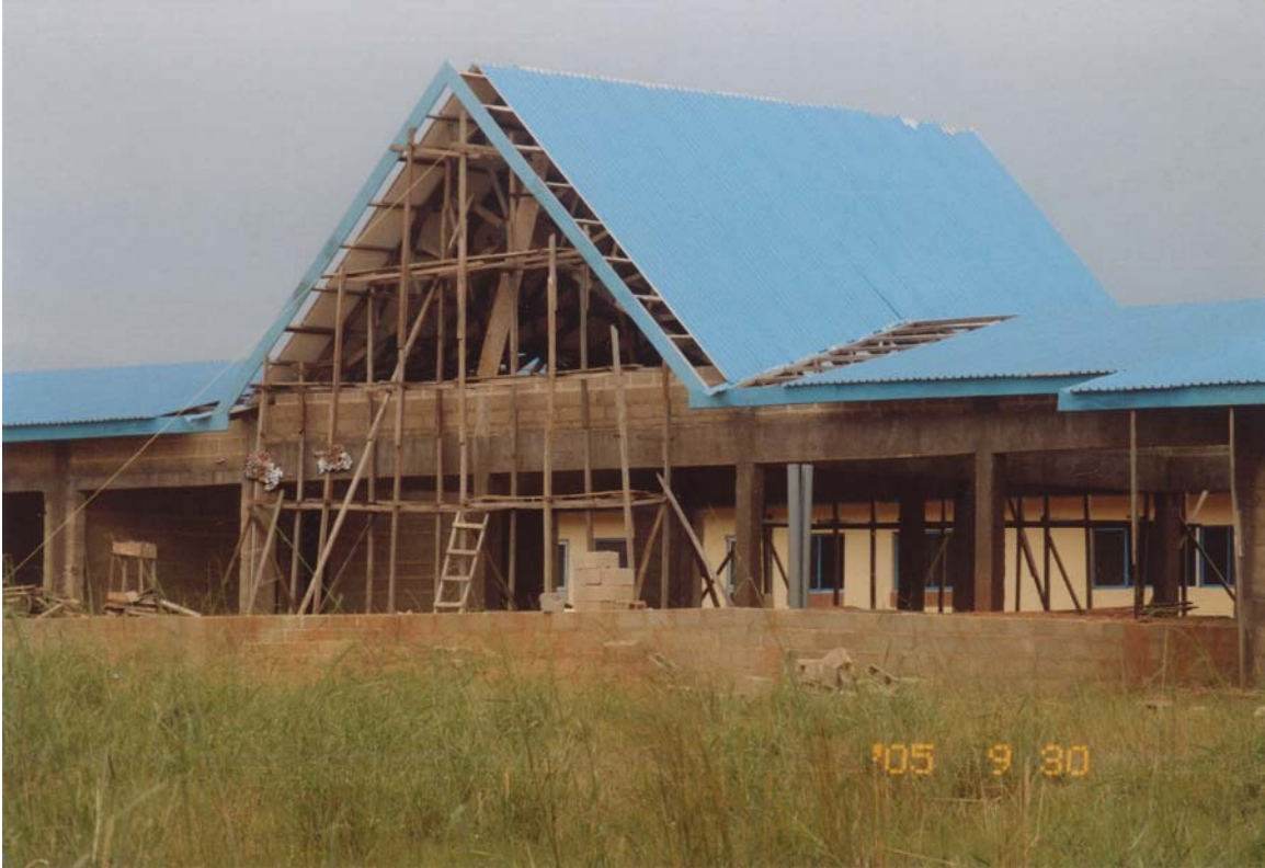
Construction at Haven of Hope. Nigeria 2005, 2006
