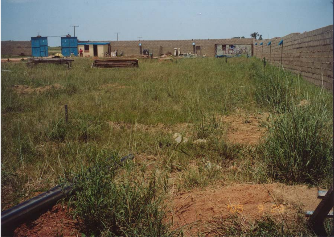
More Construction at Haven of Hope. Nigeria 2005, 2006
